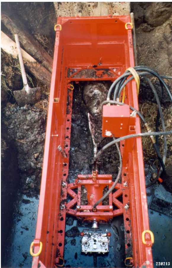
Picture left: The PE pipe has arrived. The main cylinder is slid to the rear of the TERRA-HYDROCRACK. Now the bursting rod, the expander cone and the PE pipe may be pulled into the HYDROCRACK easily.
