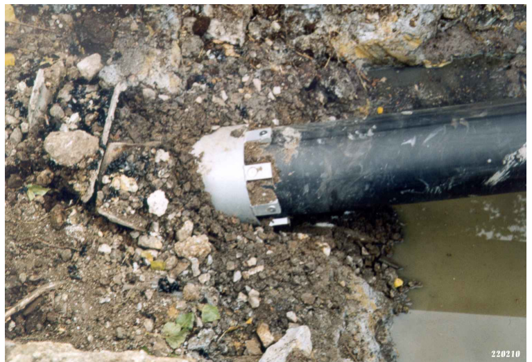
Picture left: The PE pipe OD 315 mm, 120 m long, the mini bursting sleeve OD 368 mm and the bursting rod 12" with 3 blades are prepared for operation.
