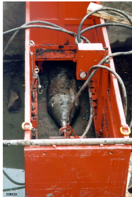
Picture below: The expander cone (mini bursting sleeve) with the PE pipe are pushed into the TERRA-HYDROCRACK. The pipe renewal project is finished
