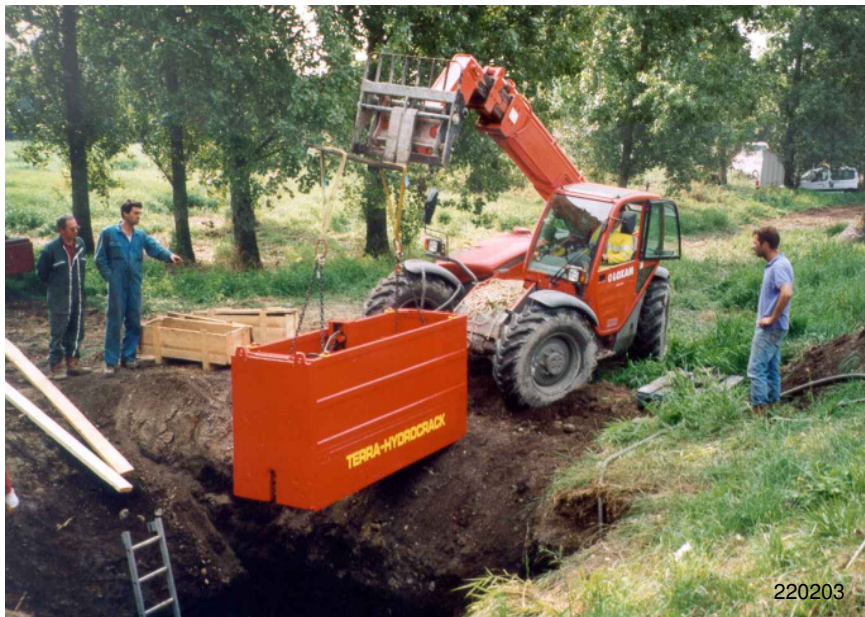
Picture left: The PE pipe OD 315 mm, 120 m long, the mini bursting sleeve OD 368 mm and the bursting rod 12" with 3 blades are prepared for operation.
