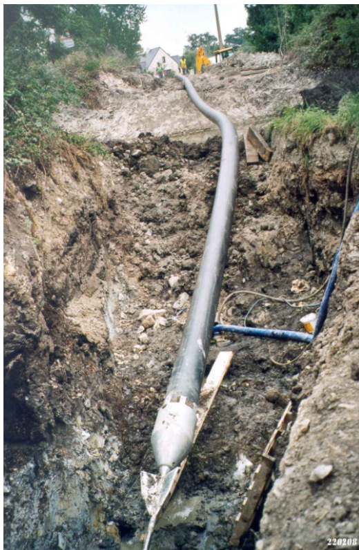
Picture left: The PE pipe OD 315 mm, 120 m long, the mini bursting sleeve OD 368 mm and the bursting rod 12" with 3 blades are prepared for operation.
