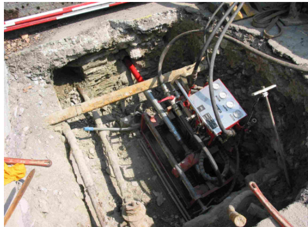
Right: The TERRA-ROCK Air Percussion Head \varnothing 65 mm during starting, now with the sonde housing.
