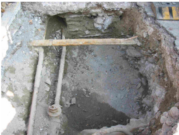
Left: A view into the starting pit.
