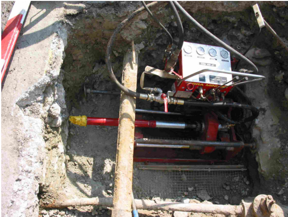
Above: The TERRA MINI-JET with the TERRA-ROCK Air Percussion Head \varnothing 65 mm. For starting the short starting adapter is used instead of the longer sonde housing.
