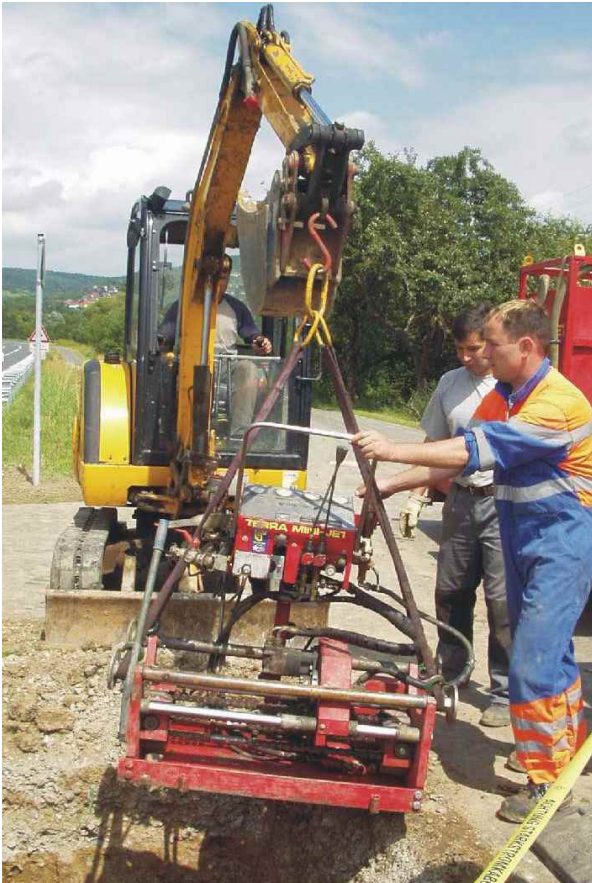
The TERRA MINI-JET is lifted into the working pit with a mini excavator.
