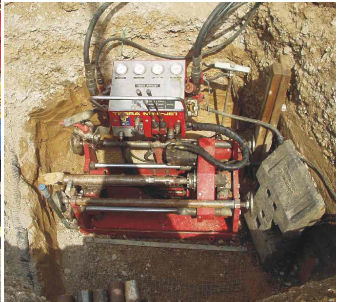
The TERRA MINI-JET is positioned in the working pit, ready for the pilot bore.
