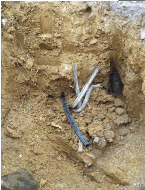
Pic. right: The HDPE pipe OD 25 mm (1") is pulled in within less than 8 minutes. The PE pipe adapter OD 25 mm (1") allows an easy connection to the new HDPE pipe.
