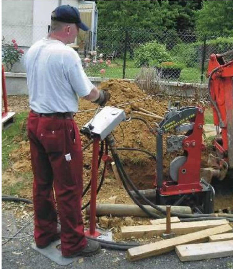
The TERRA-EXTRACTOR X 100 in the working pit. The operator stands besides the pit and controls the wire burster with the control station.
