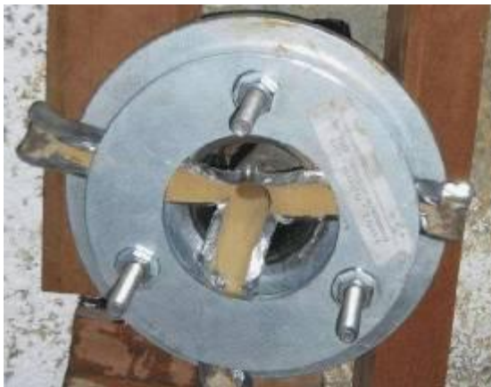
The beginning of the old lead pipe in the cellar is cut into 3 slices and fixed with the patented blocking system.
