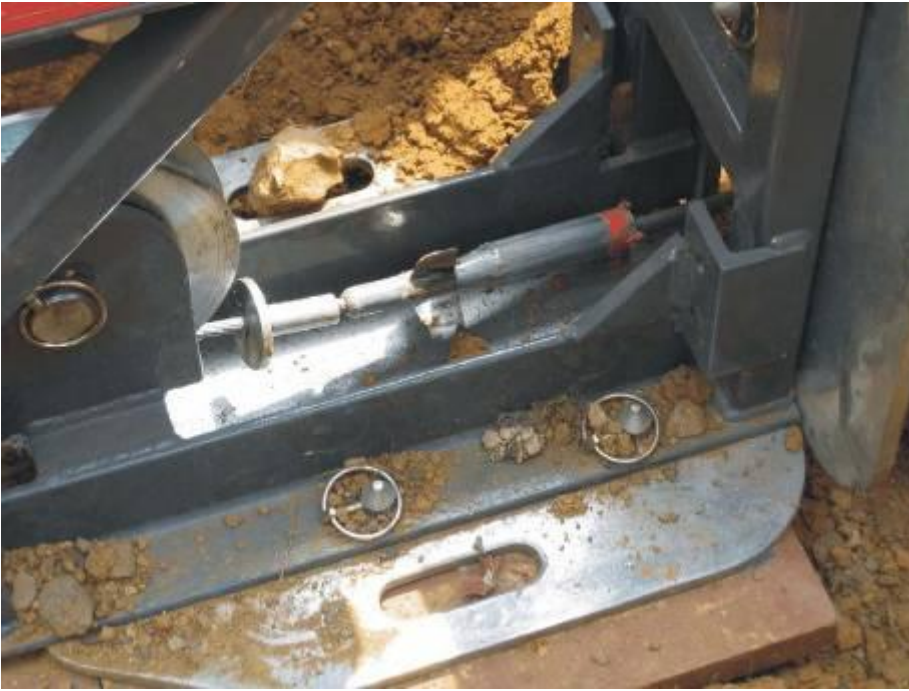
Pic. left: 12 m of old lead pipe are cut after 15 m (40 ft) minutes. Then the second pulling cable \varnothing 8 mm (0.3") can be pulled in together with the connected HDPE pipe OD 25 mm (1").
