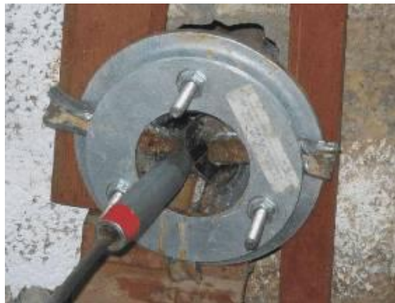
Then the 3-wing-cutter cuts the lead pipe easily with low cutting forces into 3 slices.
