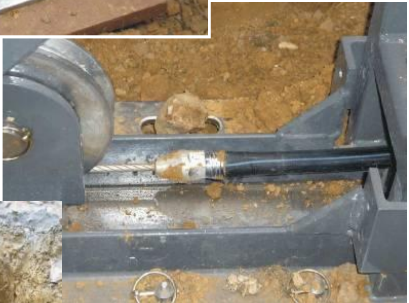
Pic. right: The HDPE pipe OD 25 mm (1") is pulled in within less than 8 minutes. The PE pipe adapter OD 25 mm (1") allows an easy connection to the new HDPE pipe.
