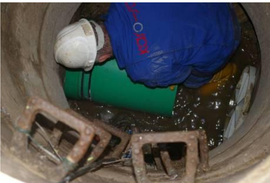
← The next pipe module is assembled.
