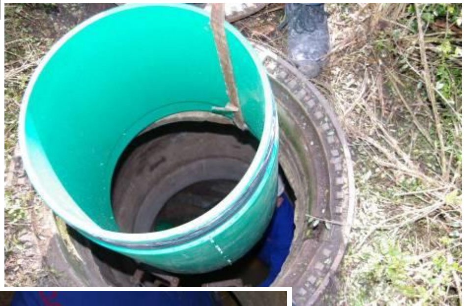
→ The next pipe module PP-HM DA 485 mm (19") is lowered into the manhole.
