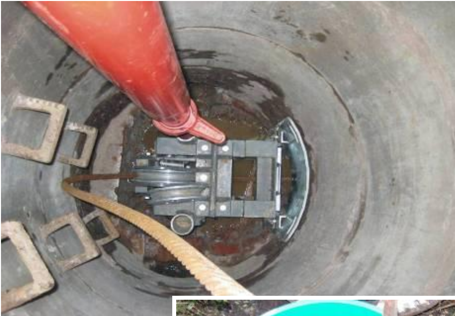
← The manhole frame, the front plate and the two struts are lifted through the opening \varnothing 62.5 cm (24.6") and assembled at the bottom of the manhole.
