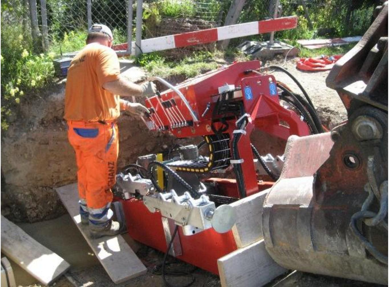
The Swiss contractor Tschanz Grabenlos AG from Luterbach has used its HDD pit machine TERRA-JET 3008 ES for a bore in Bibrist. This difficult bore runs underneath existing stairs with an inclination of 48 % downwards. The pit machine was installed in the starting pit with this inclination.
