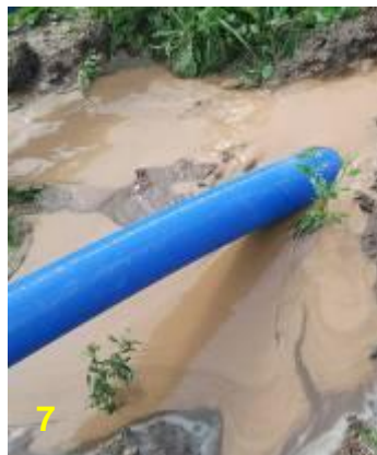
7 The HDPE pipe is pulled in. The drill mud continuously flows backwards
