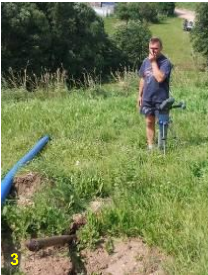
3 The drill head reaches the target point exactly in the part of the new waterline.
