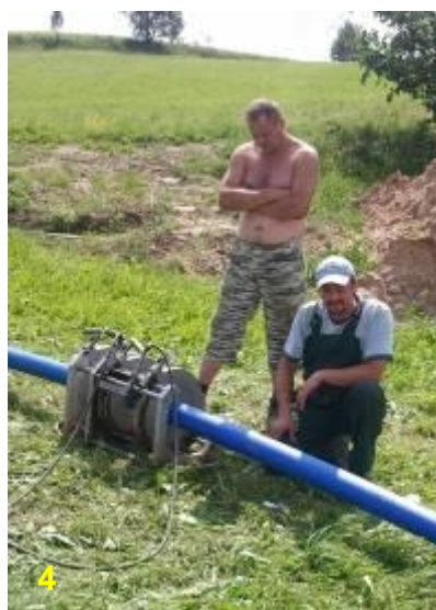
4 Butt fusion of the HDPE pipe OD 110 mm (4.3").
