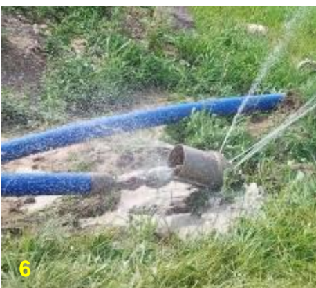
6 The backreaming begins. Bentonite comes out of the jet nozzles of the backreamer.
