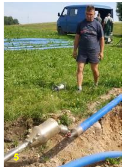
5 The backreamer OD 260 mm (10") with 130 m (425 ft) of HDPE pipe OD 110 mm are assembled.
