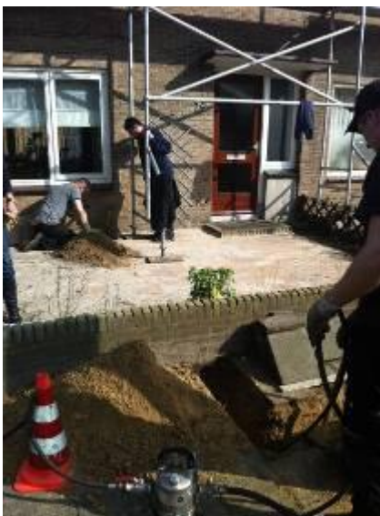
← The TERRA-HAMMER T 055 SK reaches the target pit after 5 minutes.
