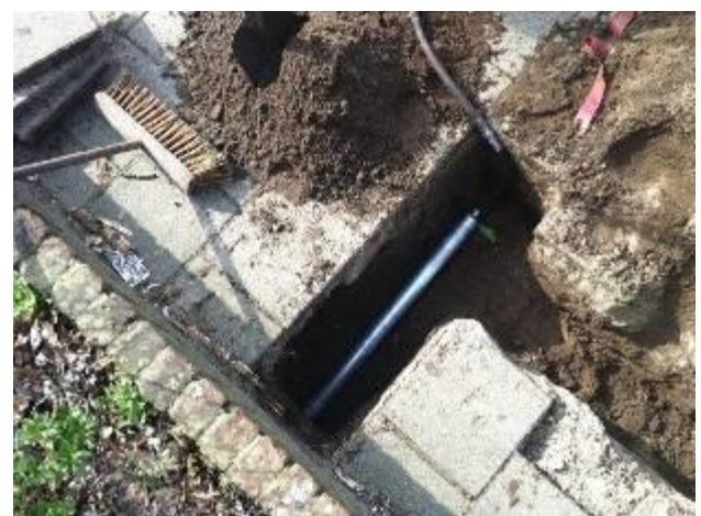
The TERRA-HAMMER T 055 SK penetrates into the ground.
