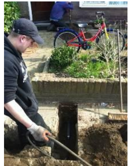
→ The TERRA-HAMMER T 055 SK has just started the bore.
