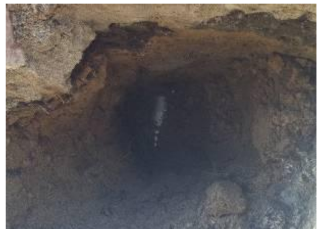
→ The TERRA-HAMMER T 055 SK has reached the arrival pit right on target.
