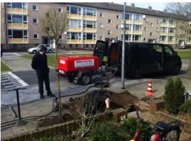
The launching pit is prepared.
