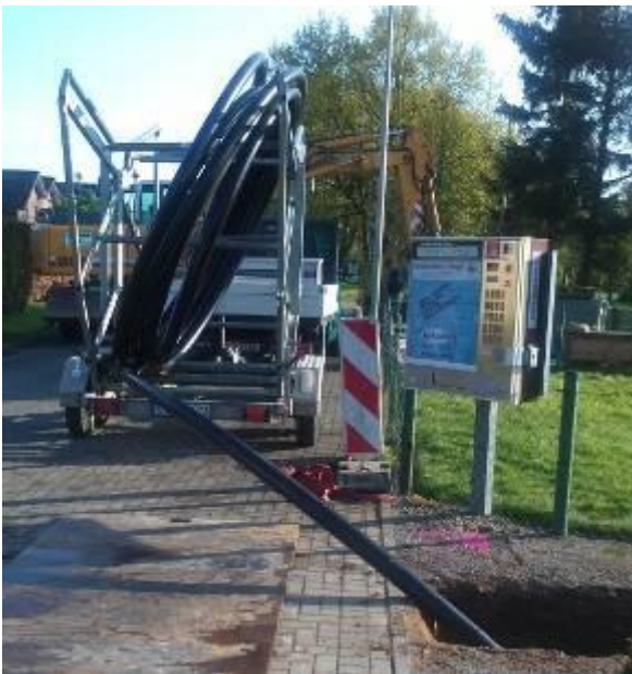
The new HDPE pipe is pulled in directly from a cable drum.
