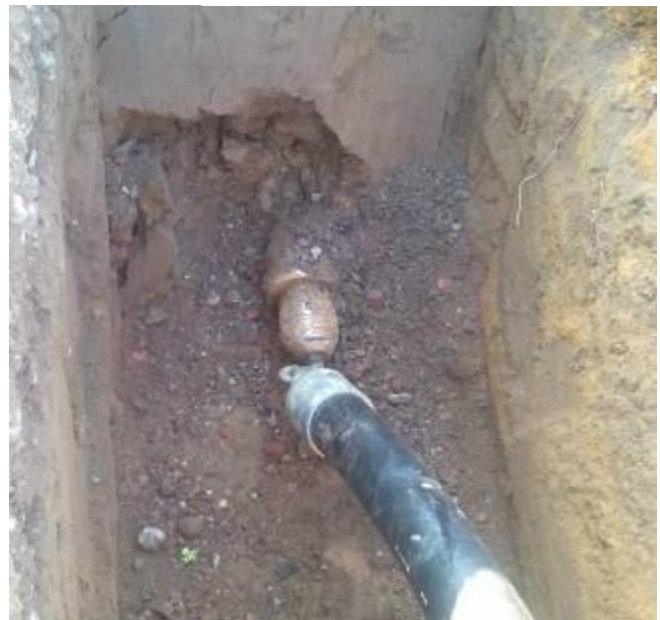
The backreamer 160 mm (6.3") with the HDPE pipe OD 110 mm (4.3") just before pipe pulling.
