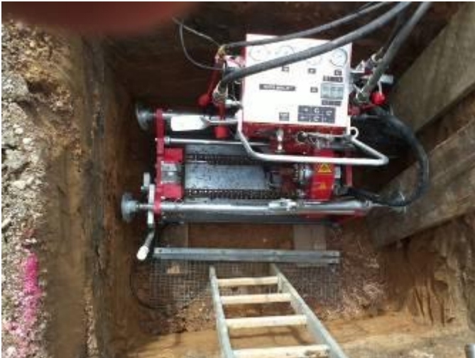
The TERRA MINI-JET MJ 1600 in the starting pit.
