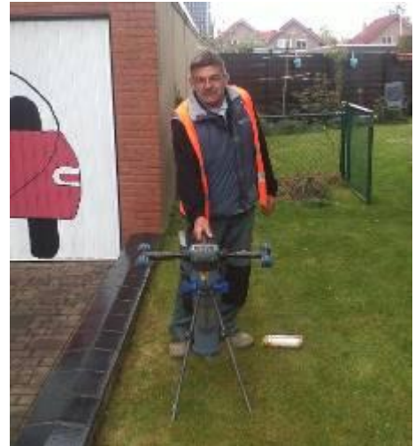
The pilot bore is located precisely with the locating system i-Track.
