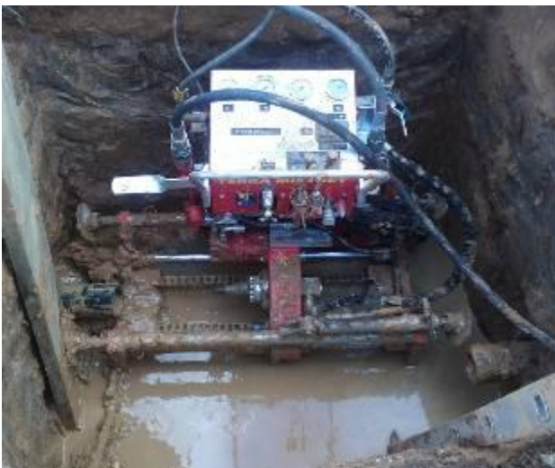
The new HDPE pipe is pulled in directly from a cable drum.
