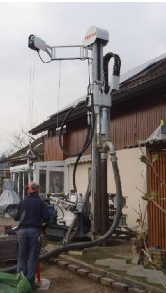
For the first 46 m (152 ft) the casings OD 152 mm (6") and the drill rods OD 89 mm (3.5") with the DTH hammer were drilled down simultaneously.
