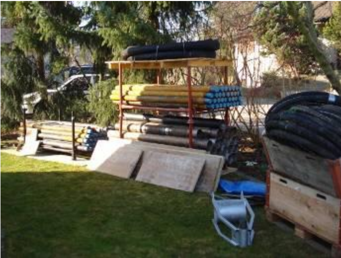
The 2 m (6.6 ft) long drill rods OD 89 mm (3.5") and the casings 152 mm (6") were stored in the front garden.
