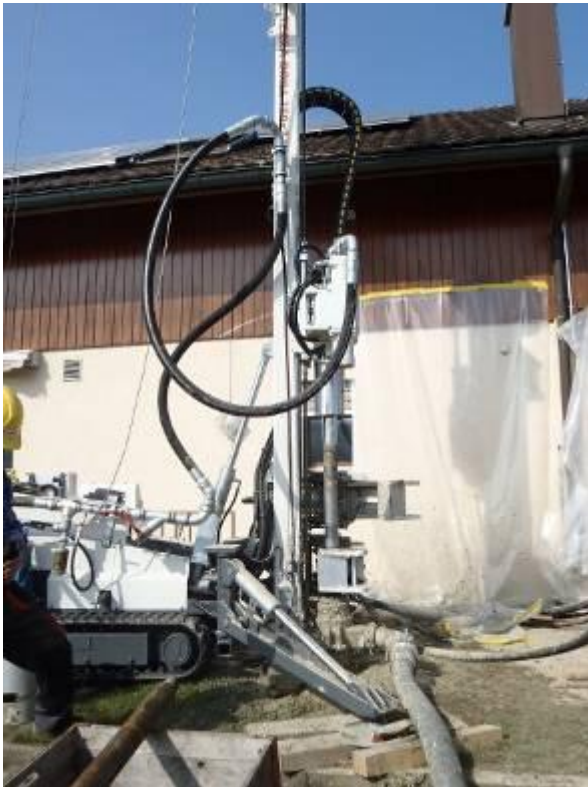
The casings are drilled down for 46 m (152 ft). The DTH hammer with the drill rods continues alone down to the final depth.
