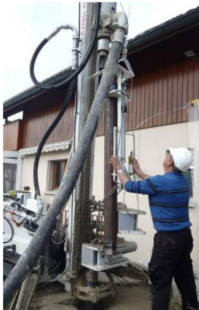
A new pair of casing pipe with inner drill rod is lifted to the drill with the handling system and hydraulically screwed on.
