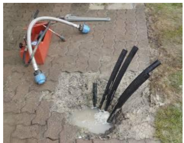
One of the two earth sondes (double-U-sonde OD 40 mm (1.57") with 25 mm (1") filling pipe) after the filling of the bore channel.
