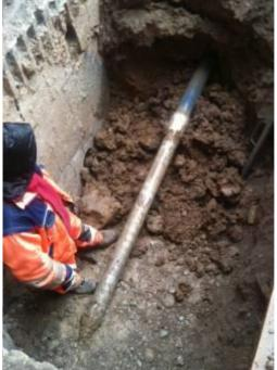
After 11 m (36 ft) the TERRA-HAMMER reaches the arrival pit right on target.
