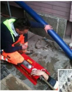
The PE pipe is pulled in simultaneously with the TERRA-HAMMER.
