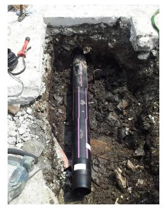
The cable burster TERRA-EXTRACTOR X 400 with a pulling forces of 400 kN (40 tons) easily pulls in the pipe stepwise.
