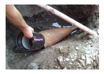
The first half-metre (19.7") short pipe module is screwed in and tightened with the strap wrench. After pull-in steps of a half-metre the further short pipe modules were threaded in.
