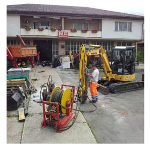
The cable burster TERRA-EXTRACTOR X 400 installed in the pulling pit. The hydraulic drive and the power supply for the machine as well as for the cable drum came from the hydraulic power take-off of a 5-to excavator.
