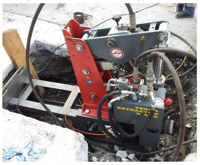
The pipe rehabilitation of a dilapidated sewer in Rothenthurm, canton of Schwyz (Switzerland) was carried out by Rudolf Frutig from Mühlethurnen, a company specialsied in berstlining. In the start pit the space was limited, therefore the choice of pipe system were threadable short pipe modules. After preparing the pits and installation of the cable burster, the pulling in of the 12 m (39 ft) pipe was executed within 30 min. This pipe went underneath a concrete slab.
