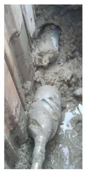
The backreamer  $\emptyset$  260 mm (10.2") is assembled in the arrival pit. The HDPE pipe OD 180 mm (7.1") is connected via an expander chuck.
