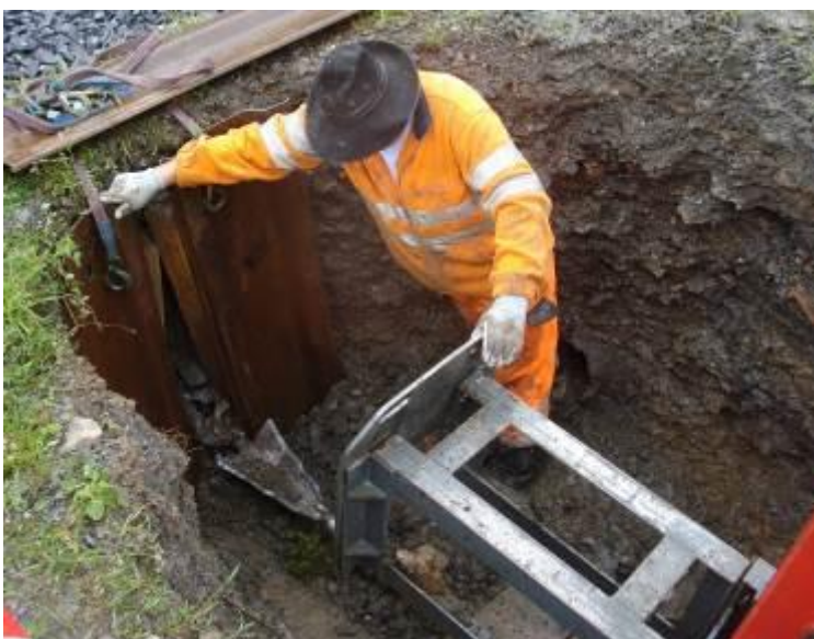
The 3-wing cutter arrives in the working pit.
