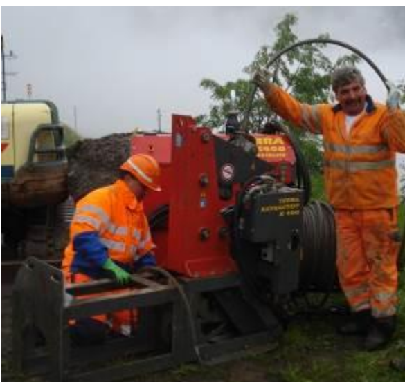
The pulling cable is slid through the cable burster and through the old pipe.
