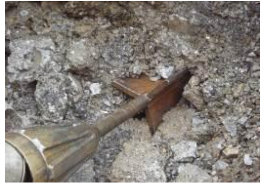
The 3-wing cutter bursts the old concrete pipe.
