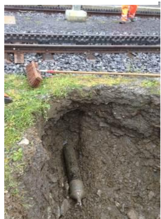
The new pipe is pulled in.
