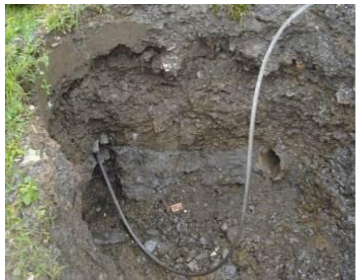
The pulling cable is slid through the cable burster and through the old pipe.
