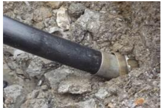
The expander cone displaces the old pipe sideways and produces a large channel for the new pipe.
