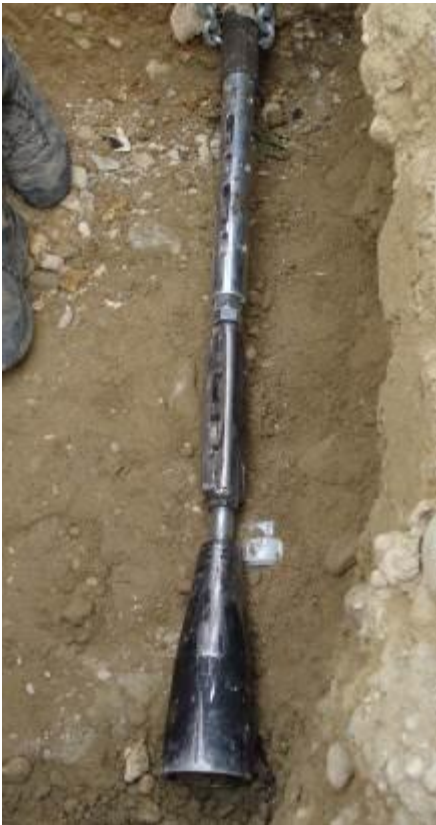
← The roller cutter is pulled into the old steel pipe. The cutting rolls begin to cut.
