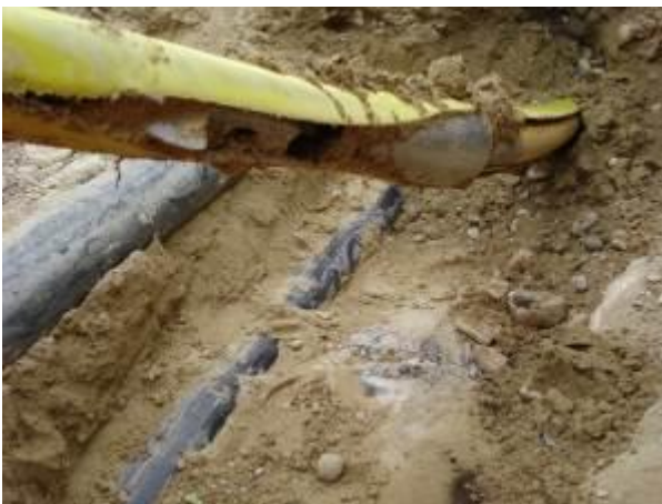
The bursting tool with the new pipe arrives in the "pulling pit".
