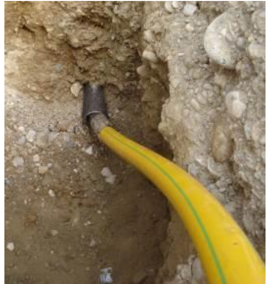
The new HDPE pipe OD 63 mm (2.5") from Simona AG is pulled in.
