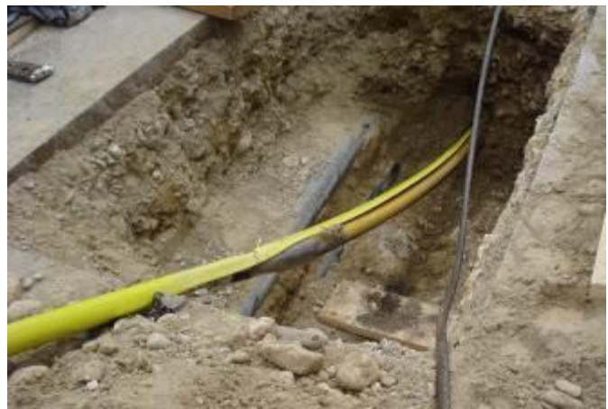
The cable burster is positioned onto the edge of the "machine pit", to pull in the new pipe in the required length.
