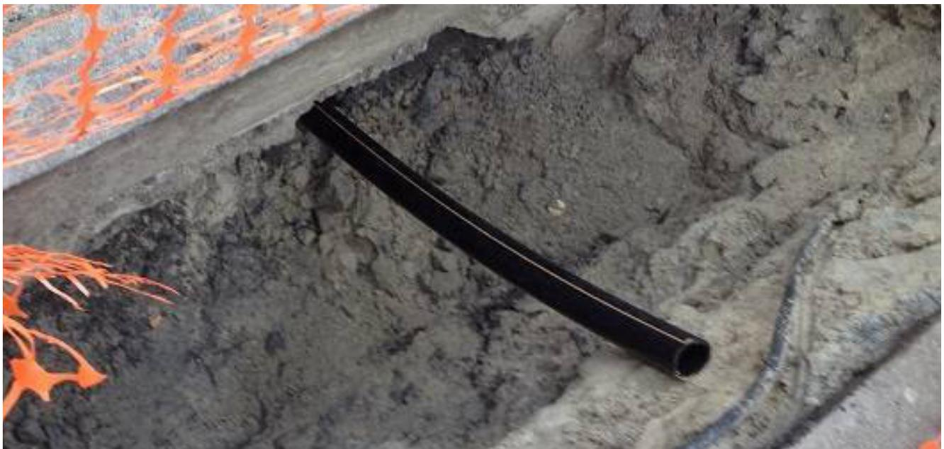
Pic. 6: The new pulled-in HDPE pipe OD 50 mm (2").
