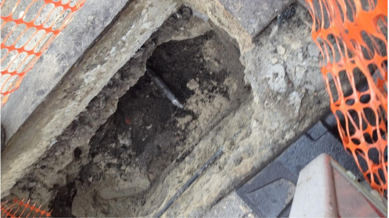
Pic. 3: Directional rod pushing allows high accuracy. The drill head reaches the arrival pit right on target.
