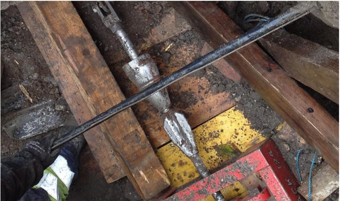
Pic. 5: The expander tools and the new pipe reach the starting pit. After only 3 working hours the jobsite with a total length of 10 m (33 ft) has been finished.
