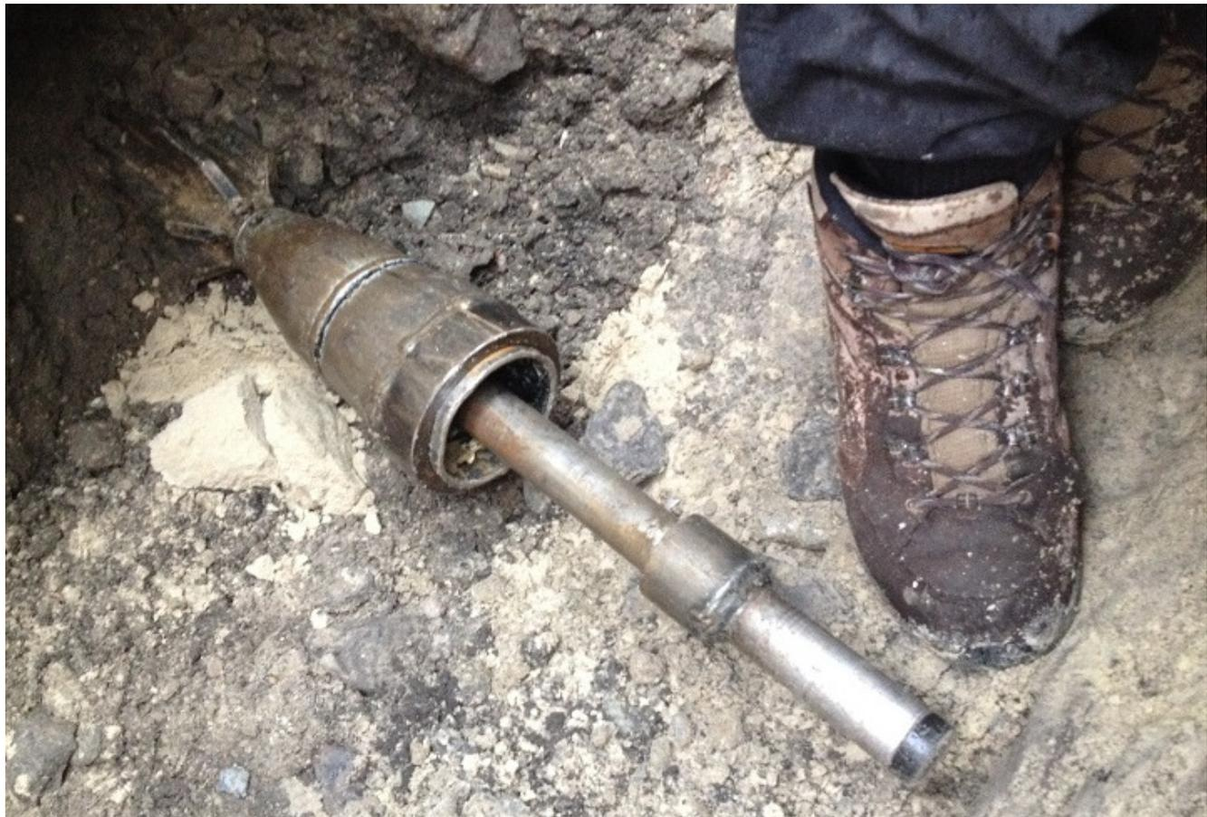
Pic. 4: After the pilot bore, the drill head is disassembled and an expander star and an expander cone are assembled. Behind comes the new HDPE pipe.
