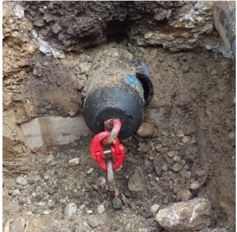
Pic 7: The new HDPE pipe OD 160 mm (6.3'') has been pulled in.
