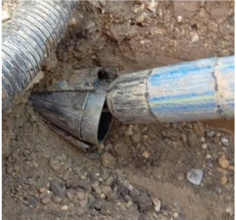
Pic 4: The Duplex PE Roller Cutter has vanished into the ground. The expander cone pushes the two halves of the old PE pipe sidewise.
