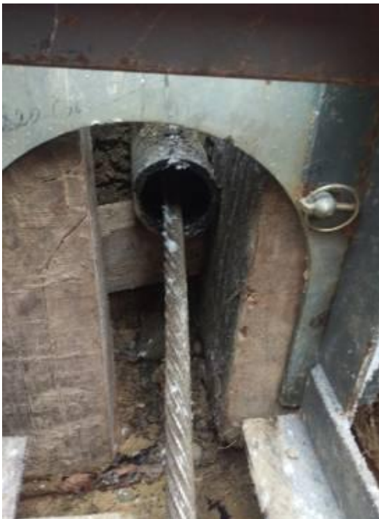
Pic 1: The pulling cable is pulled through the old pipe.
