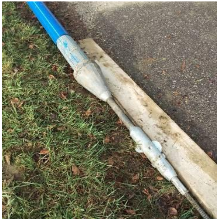
Pic 2: At the other end of the pulling cable the Duplex PE Roller Cutter, the expander cone and the new pipe are assembled.
