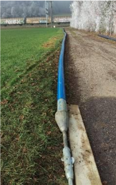
Pic 3: The new HDPE pipe OD 160 mm (6.3") is ready to be pulled in.
