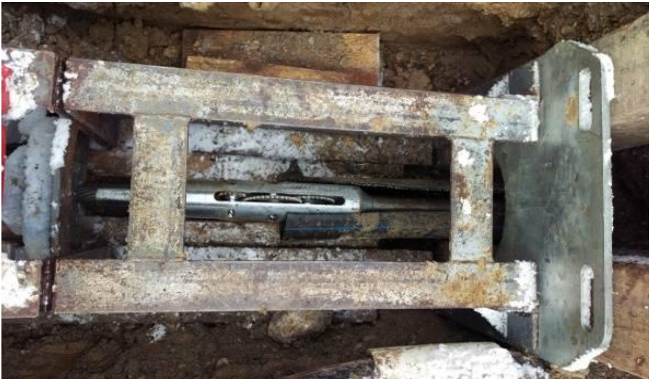
Pic 5: The Duplex PE Roller Cutter arrives in the machine pit. It has cut the old pipe clearly into two halves.
