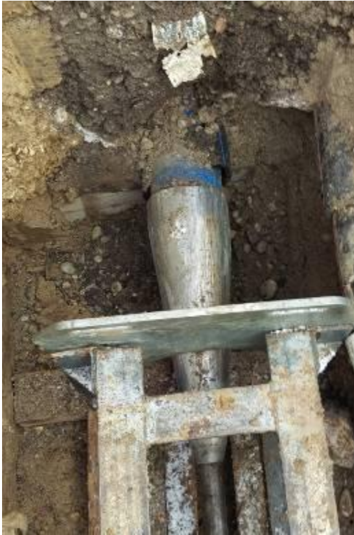
Pic 6: Expander cone and new pipe in the machine pit.
