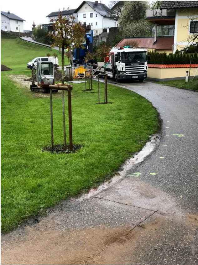
Pic 3: Drill rods allow a bending radius of 24 m.
