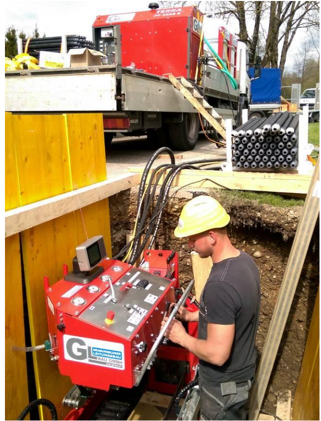
Pic 4: Drill master Thomas doing the pilot bore gradually steered on the total length of 42 m.
