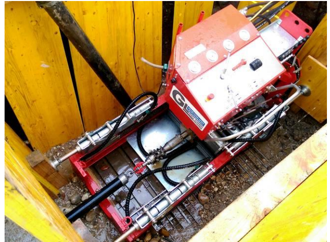
Pic 7: The pressure water pipe 90 mm was quickly pulled in with the TJ 3008 ES.
