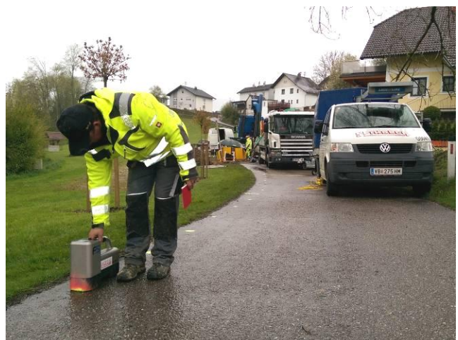
Pic 5: Foreman Markus locating the drill head with the DigiTrak F5.
