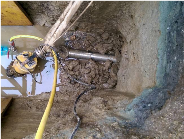
Pic 6: Accurate reach of the drill head in the target pit after the pilot bore.
