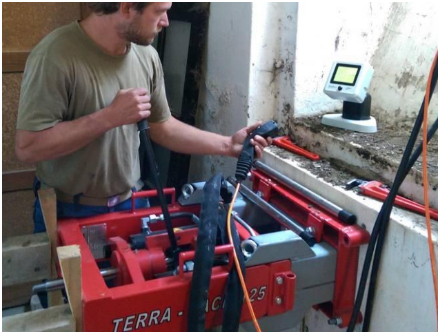
Pic 1: Drill master Ivan Isch pressing the steered pilot bore from the basement with the TERRA-JACK flanged to the wall.
