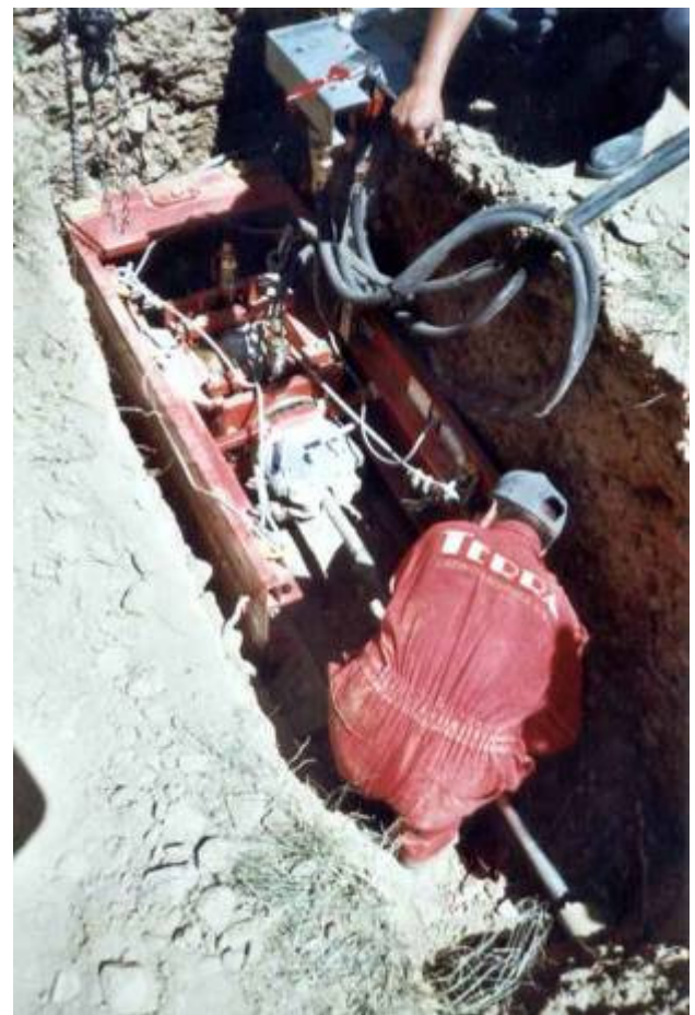
Picture above right: View onto the 100 m long job site.
