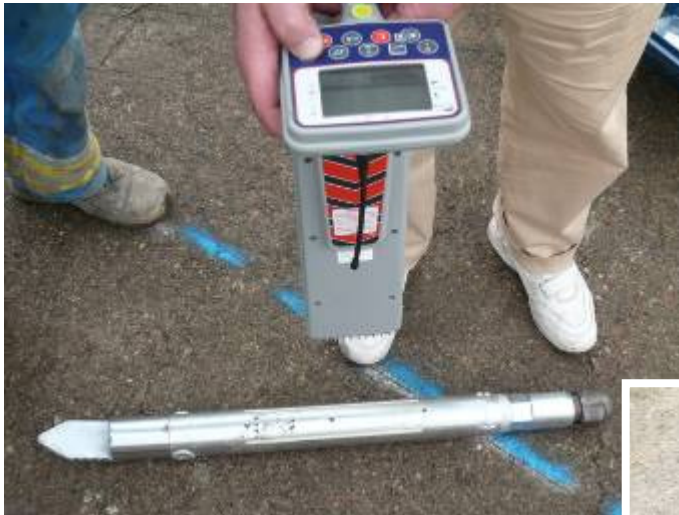
← The locator is calibrated just before the pilot bore.
