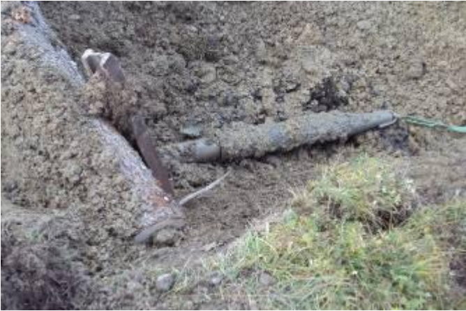
The TERRA-HAMMER with the expander and the new HDPE pipe reach the arrival pit.
