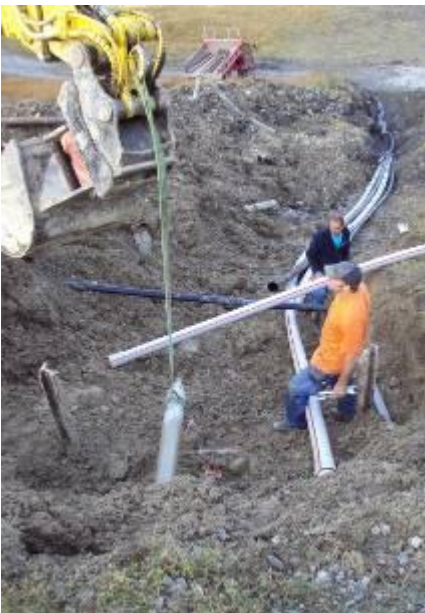
The TERRA-HAMMER with the expander and the new HDPE pipe reach the arrival pit.
