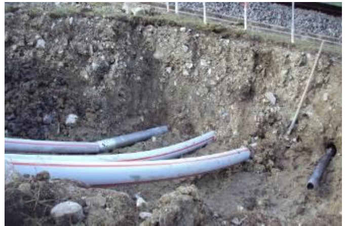
The first three pipes are laid. The TERRA-HAMMER is prepared for the forth crossing.
