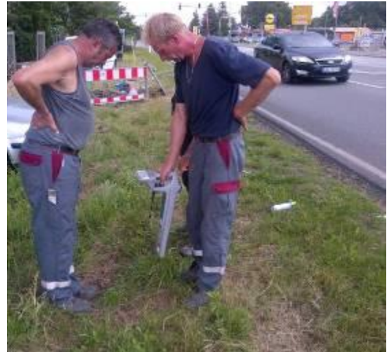
The drill head is located exactly during the pilot bore.
