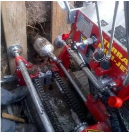
The pipe is pulled in, the bore is finished.
