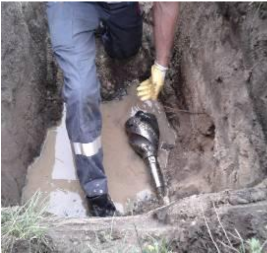
The backreamer OD 160 mm (6") is assembled. The pipe pulling may begin.
