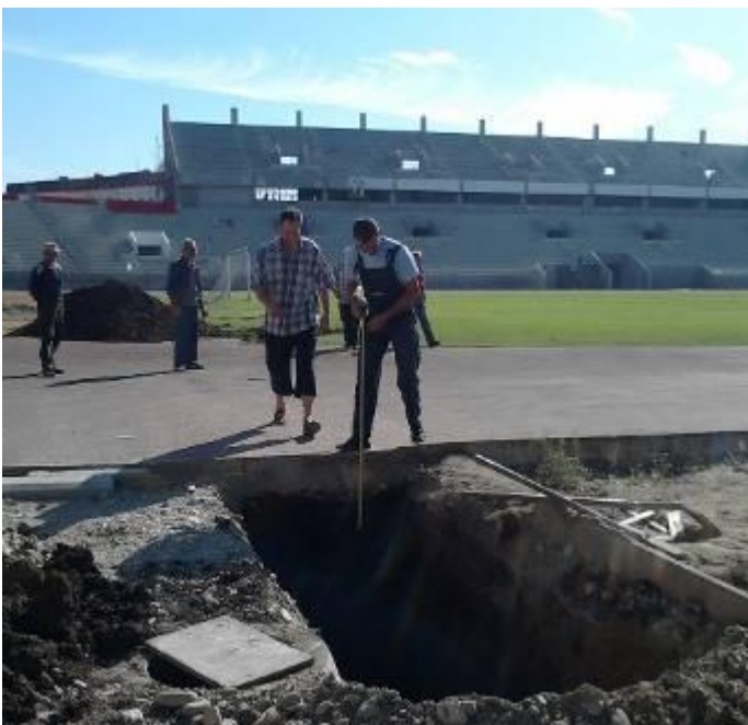
The starting and arrival pit of the first bore are prepared.
