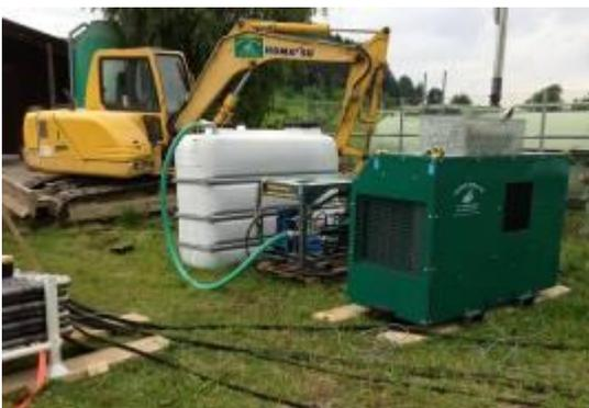
The hydraulic power pack, the mixing + pumping station as well as the tank were installed separately. The power pack is driven by a PERKINS Diesel engine. Built-on is a diesel particulate filter that ensures compliance with the strict Swiss exhaust emission standards.
