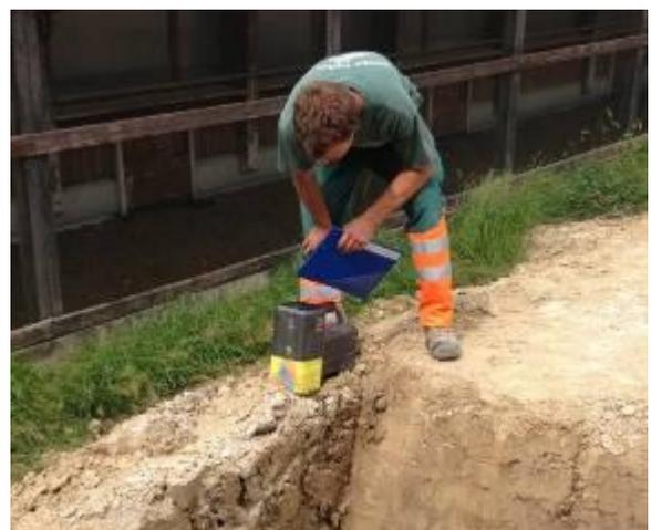
The bore run was continuously tracked with a locating system which also incorporates the target-in-the-box locating function.
