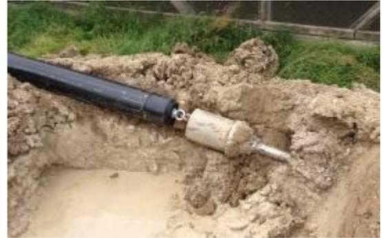
↑ The backreamer  $\varnothing$  300 mm (12") with attached HDPE pipe  $\varnothing$  225 mm (9").
