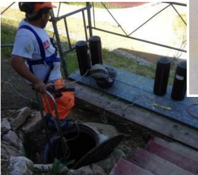
← After the pilot bore was finished, a temporary wooden floor was built into the manhole.
