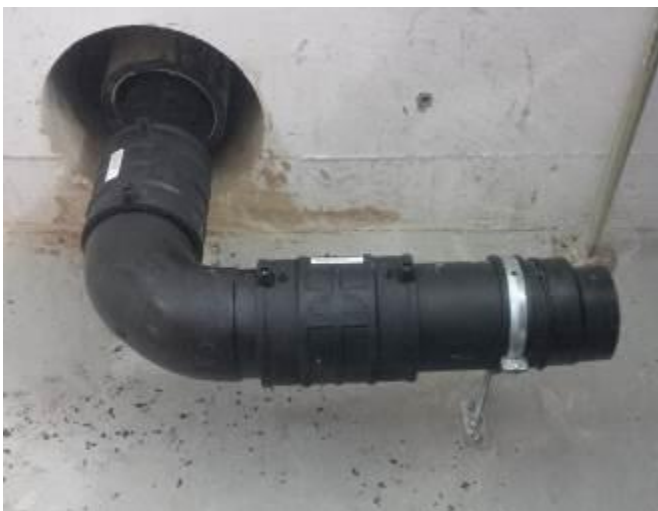
← The product pipe is assembled.
