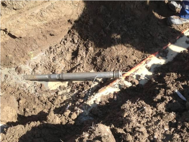
The pilot bore has been finished and arrived dead on target in the pit with the existing mainline. A 3-finger head was used as a drill head.
