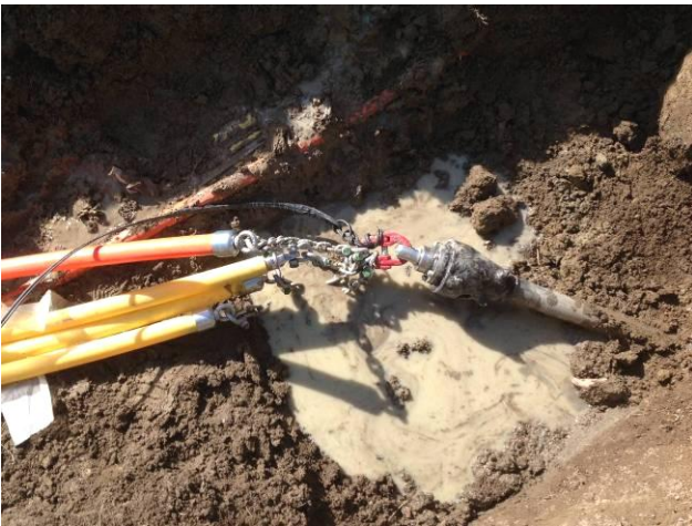
The pilot bore has been finished and arrived dead on target in the pit with the existing mainline. A 3-finger head was used as a drill head.
