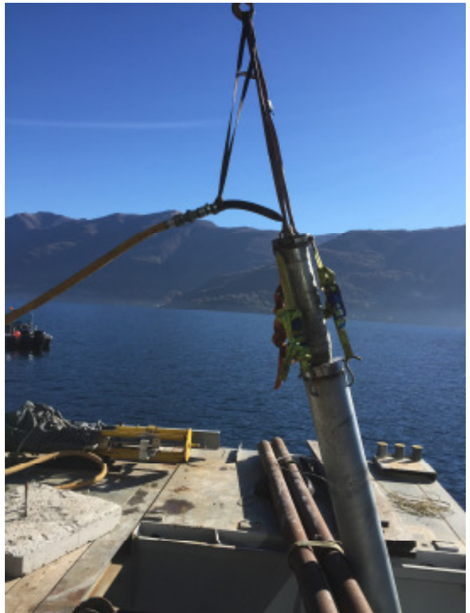
Pic. 3: The complete unit is lifted with the crane.
