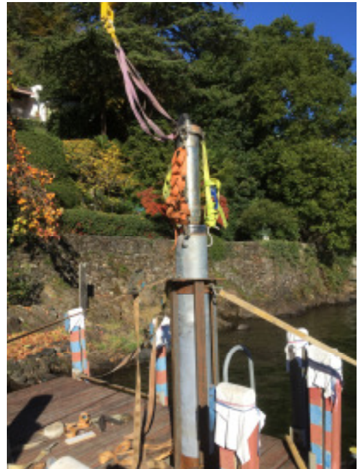
Pic. 5: The TR 200mini during ramming operation.
